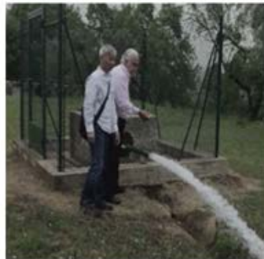
Pump Installation & Handing Over
